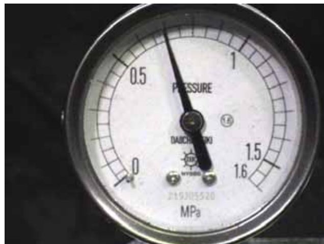
Test pressure 0.7 MPa. No pressure drop.
